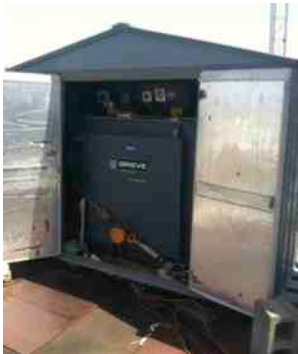
Pressurized Ovens on the Roof of the Van Leer Bldg., Ga Tech
